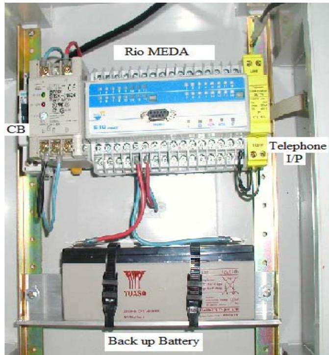
Fig. 5: Data logger Components
