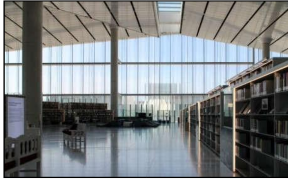
Figure 2-18: Aluminum ceiling and marble floors
