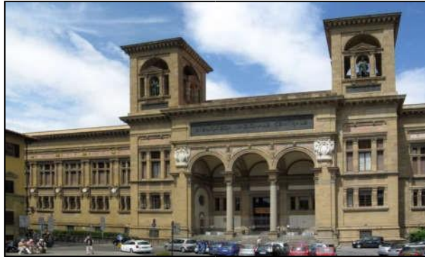
Figure 1-3: National Central Library in Florence.
