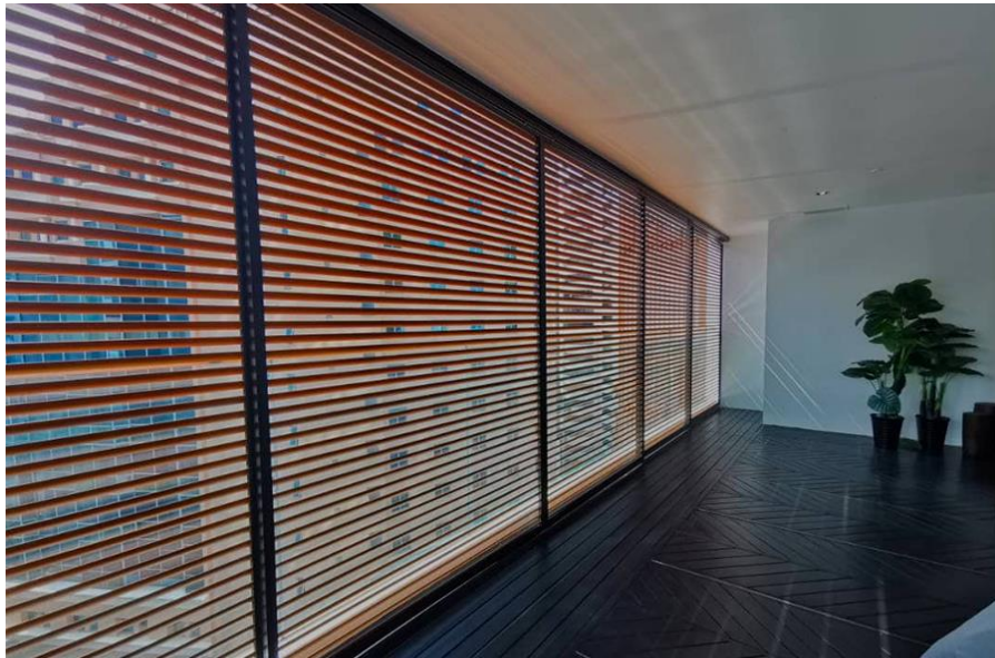
Figure 49 : horizontal window shutters
