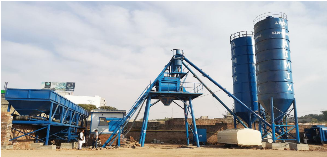
Figure 4: Wet mix concrete plant
