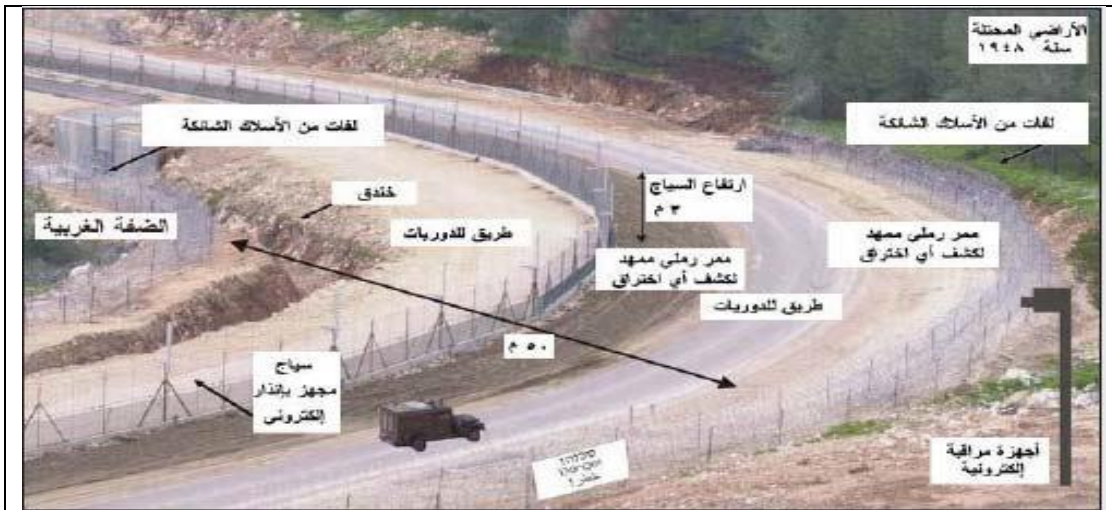
Picture(10): A cross section describing the components of the separation wall generally on west bank
