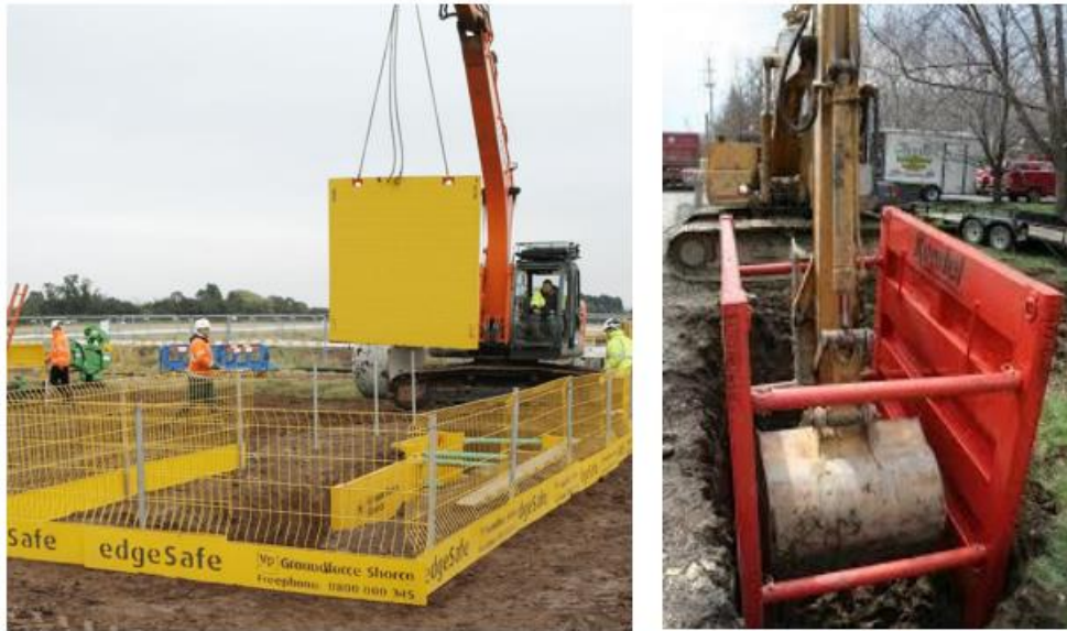
Figure 4.4: Shows Construction Machinery Excavation Compliant with All the Requirements
