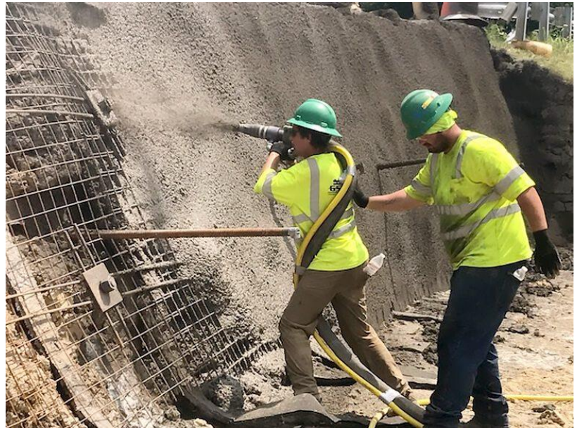
Figure 2.2: Shows the Application of Shotcrete
