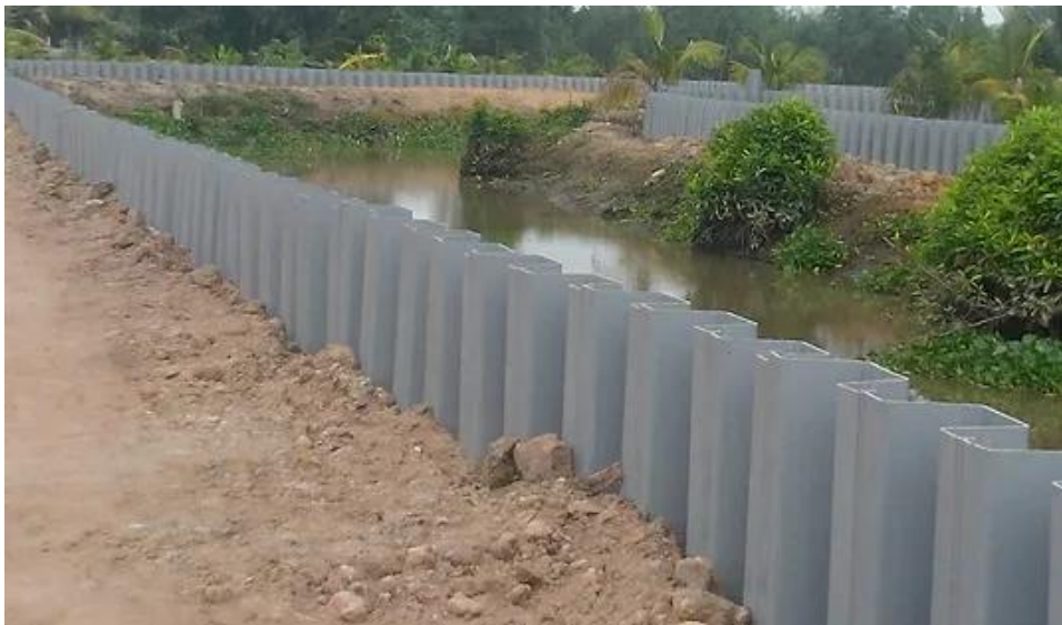
Figure 2.4: Shows the Vinyl Sheet Piles
