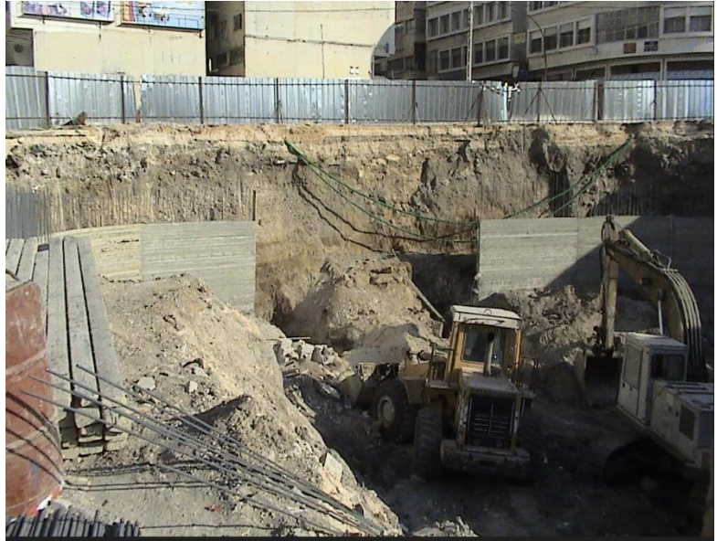
Figure 2.21: Shows a Retaining Wall of several slides
