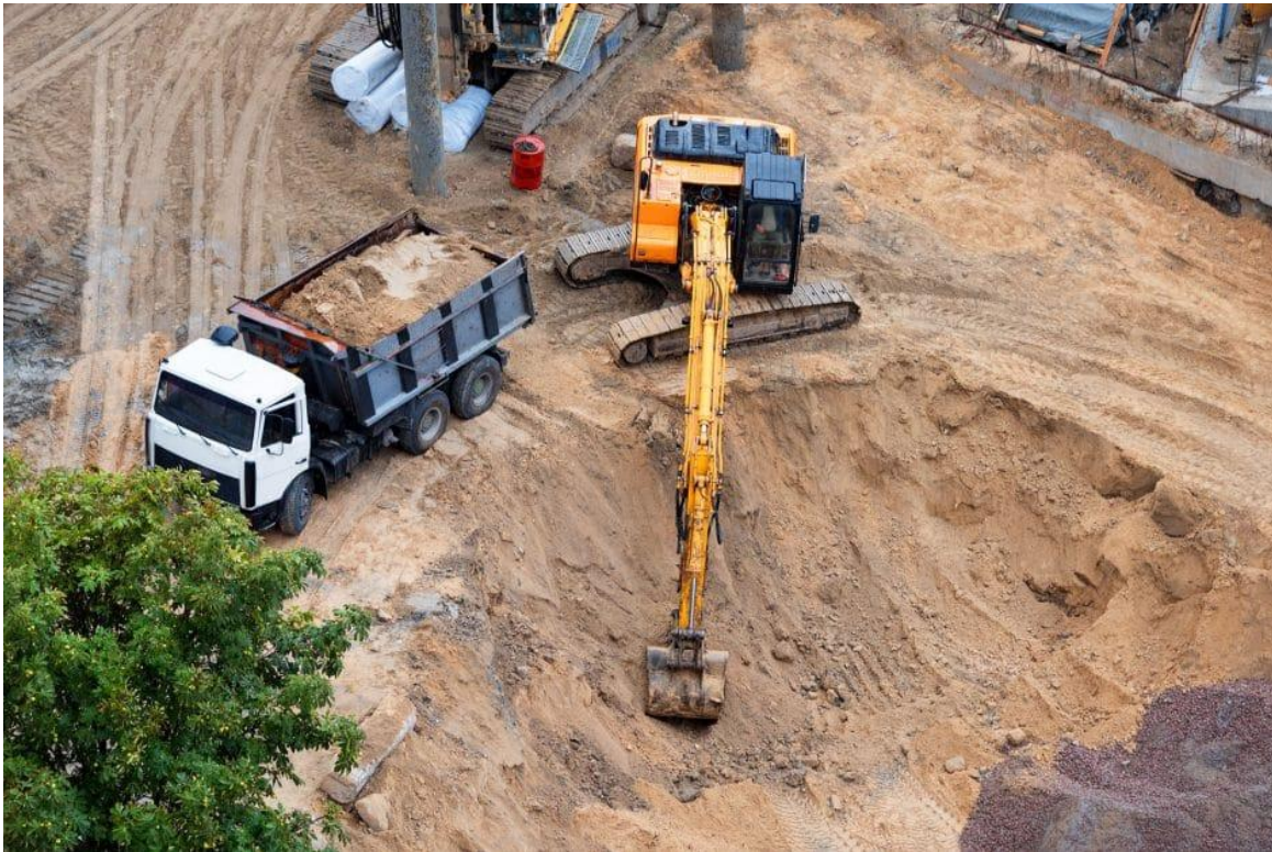
Figure 2.17: Shows Excavation without Supporting System
