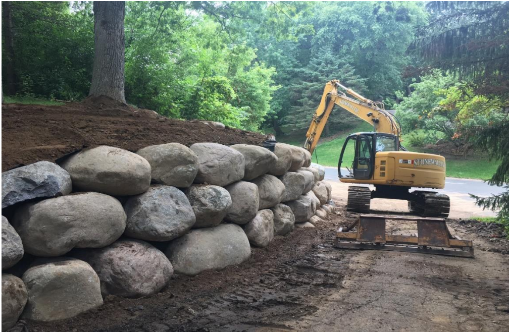
Figure 2.19: Shows the Installation of Big Boulders
