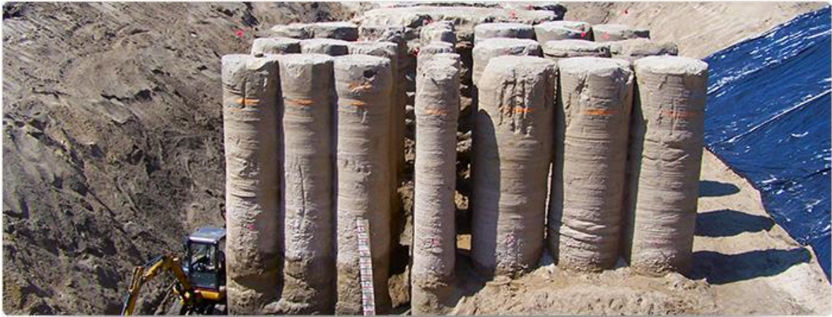
Figure 2.7: Shows Deep Soil Mixing
