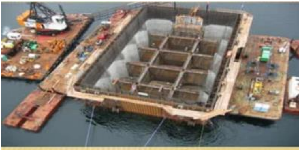
Figure 2.14: Shows the Installation of Caissons
