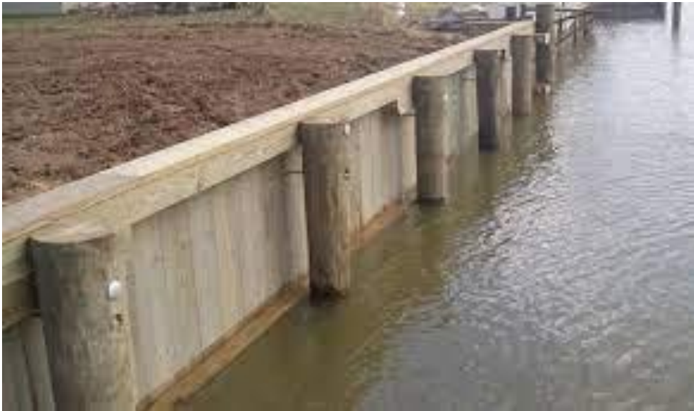
Figure 2.5: Shows a Picture of Wooden Sheet Piles
