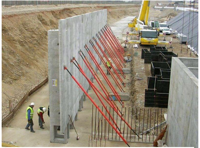
Figure 2.6: Shows the construction Process of the Concrete Sheet Piles
