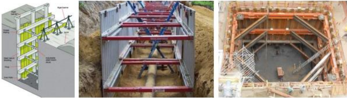
Figure 4.3: Shoring with propped formwork
