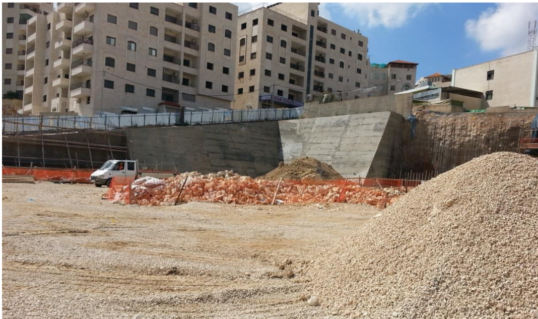
Figure 2.18: Shows a Gravity Retaining Wall
