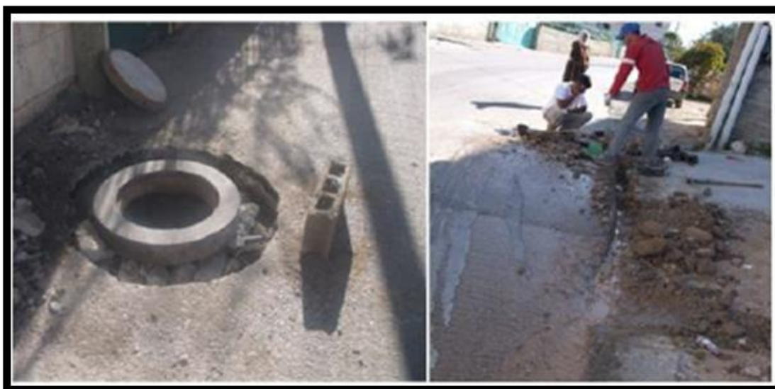
Pictures for the condition of sewage network of study area.
