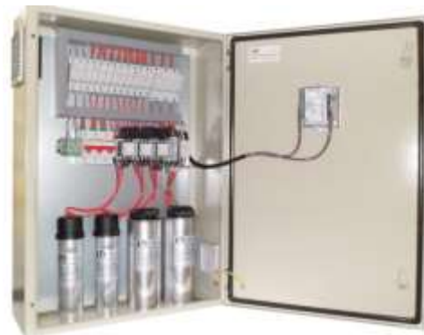
Figure 3: Automatic capacitor bank for power factor correction
