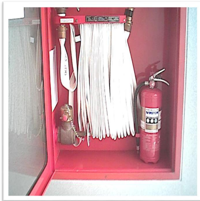
Figure 7-7: Fire hose cabinate.
