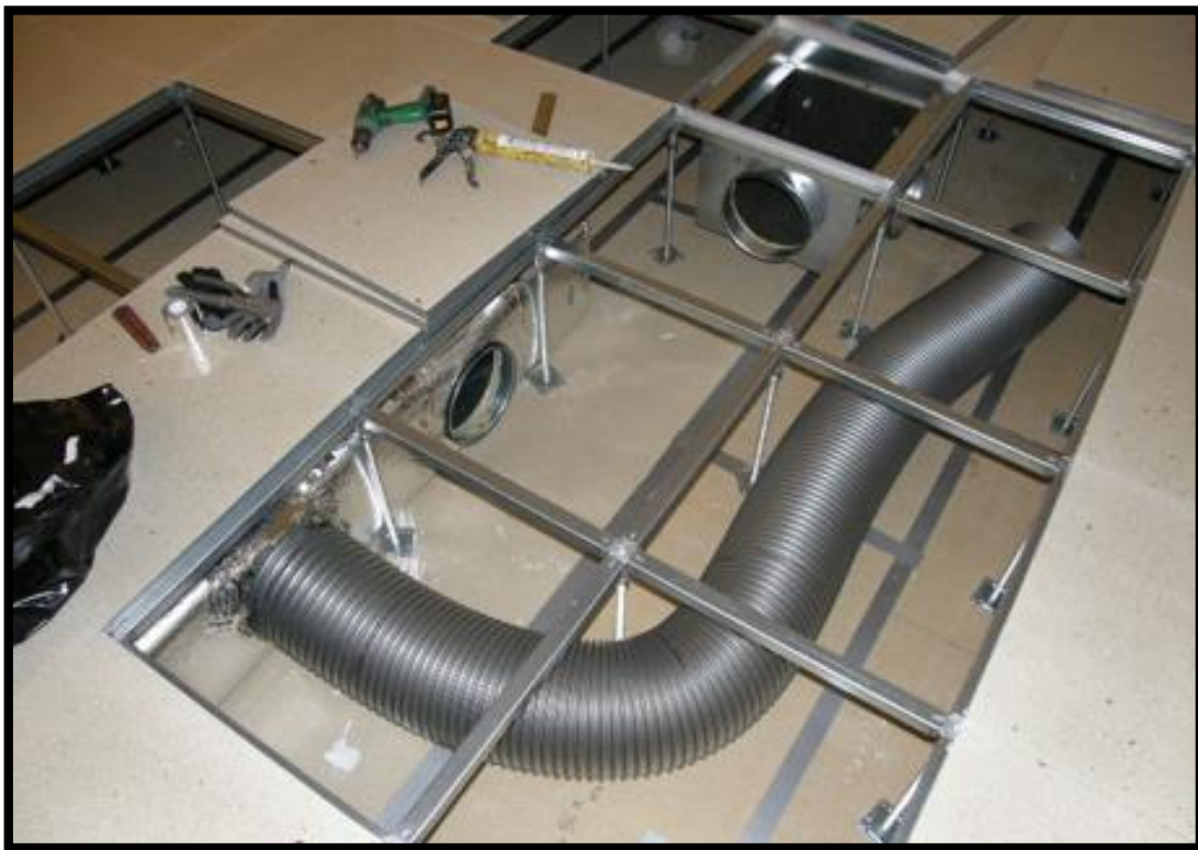
Figure 7-4 : installing HVAV under raised floor
