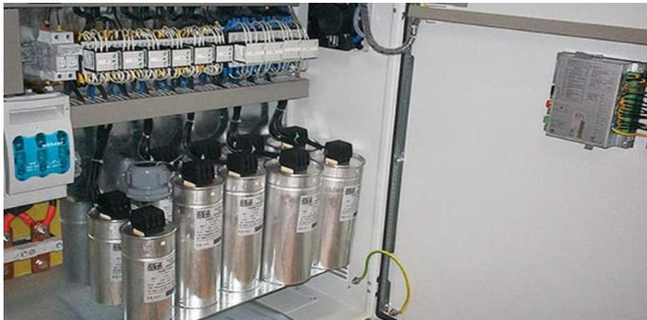
Figure 10: Capacitor banks.
