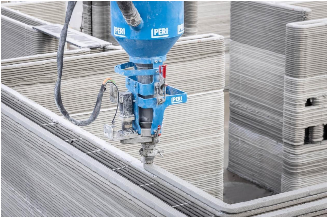
Figure 11: building 3D printed concrete house
