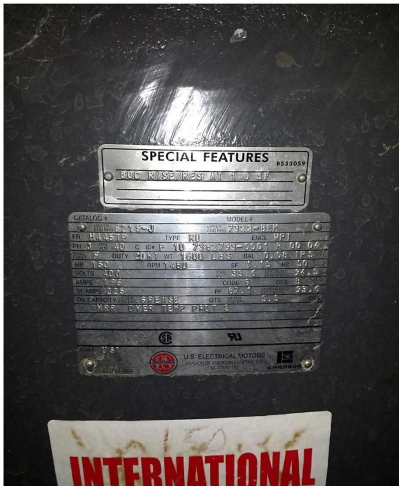
**Figure (5.12) :Name plate of Agriculture Company well motor**
