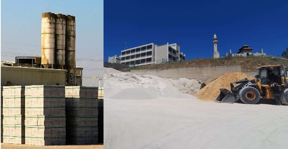
An-Najah block factory's silo and stock pile for aggregates
