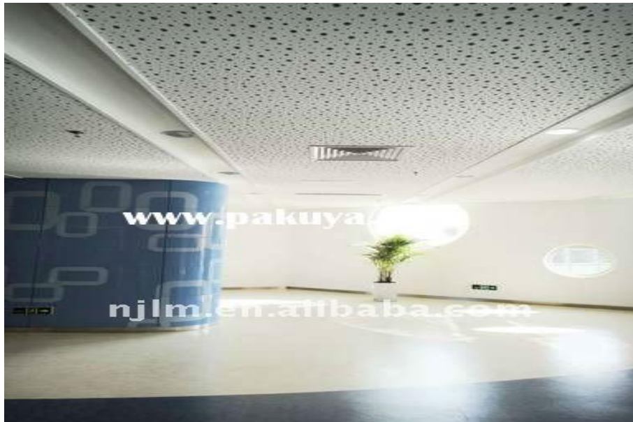
Figure 6. 16 Ceiling with perforated gypsum board.
