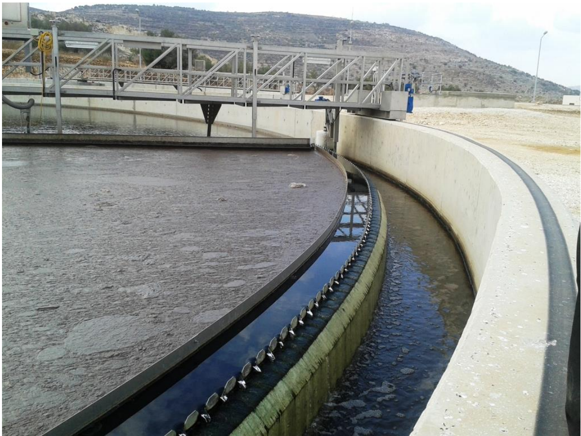
Figure 2.11: Primary Sedimentation Reservoir
