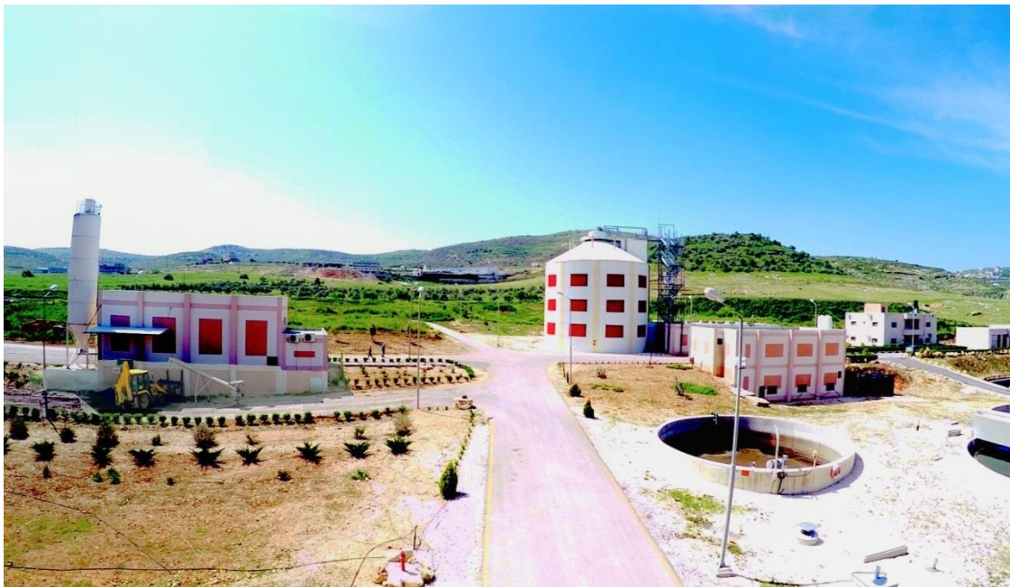
Figure 2.8: Biogas facilities ( Digester , Boiler and CHP room , sludge dewatering, biogas holder).
