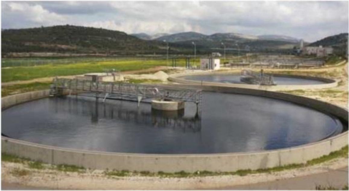
Figure 2.12 : Secondary Sedimentation Reservoir
