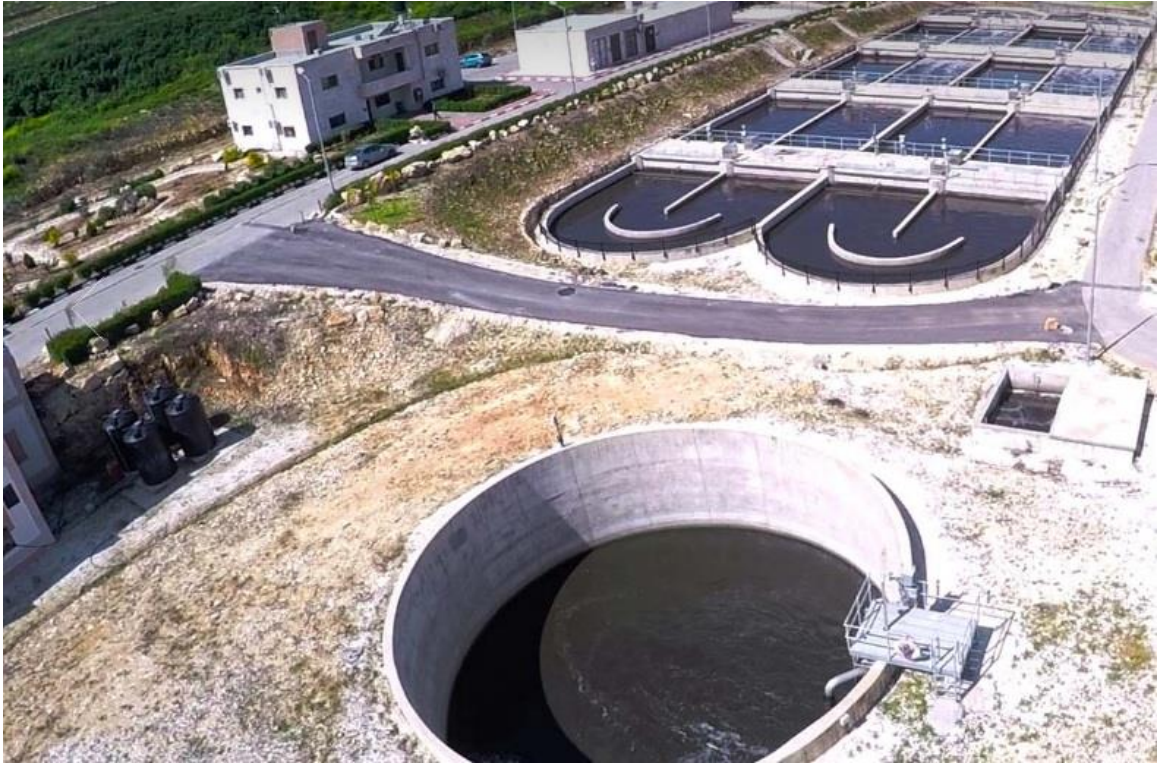
Figure 2.11: Primary Sedimentation Reservoir
