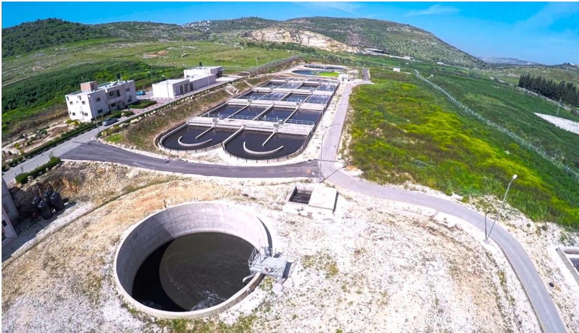
Figure 2.7: General view of treatment facility
