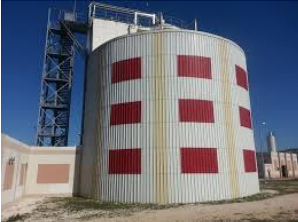
Figure 2.9: Anaerobic Digester
