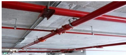
Figure 168 sprinkler pipes
