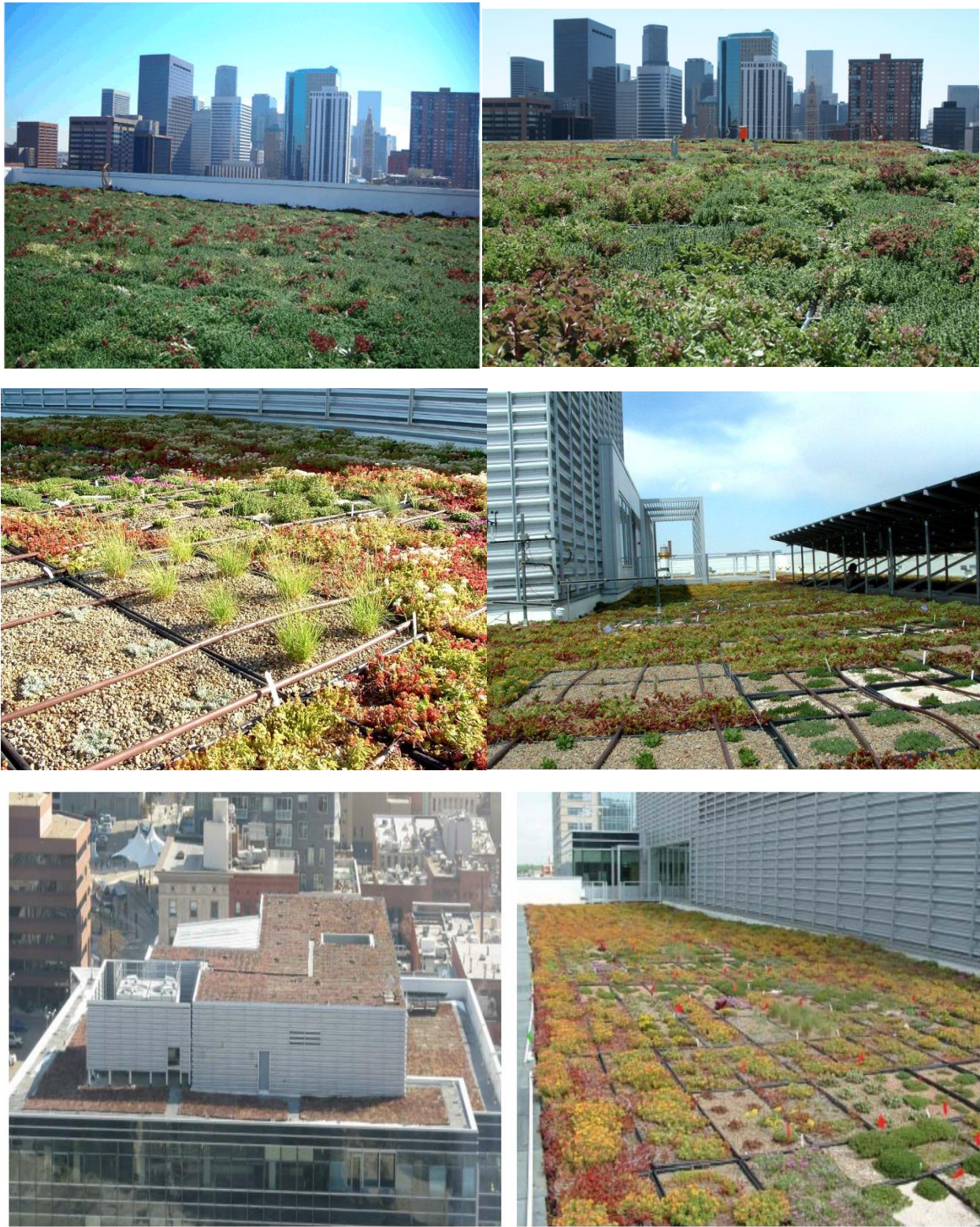
Figure 182 Pictures of EPA project [29]
