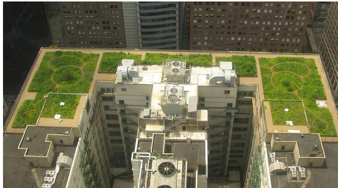
Figure 178 Chicago City Hall Green Roof
