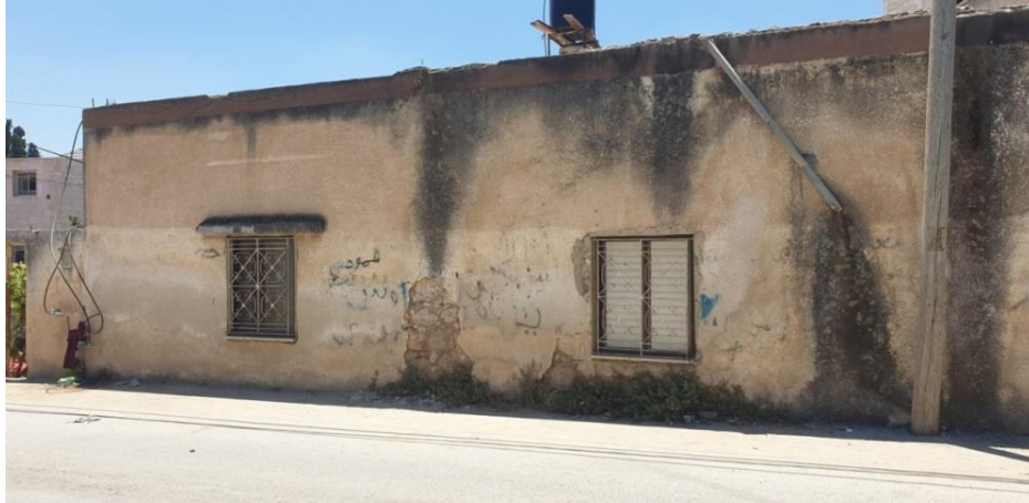
Figure 4. 32 shutter aluminum windows, and sliding aluminum glass windows barred with protective iron railing
