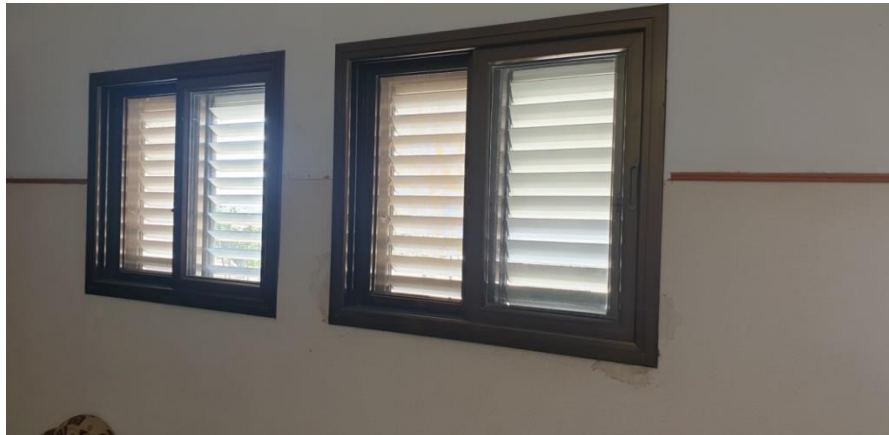
Figure 4.34 newly added Aluminum windows
