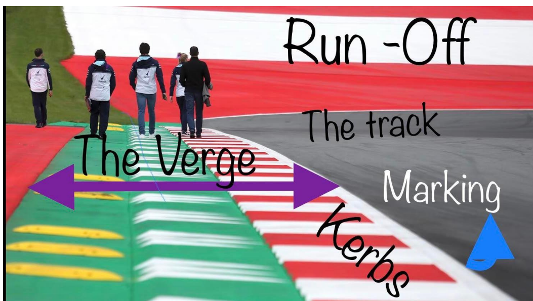
Figure 4.23: Track Side Marking
