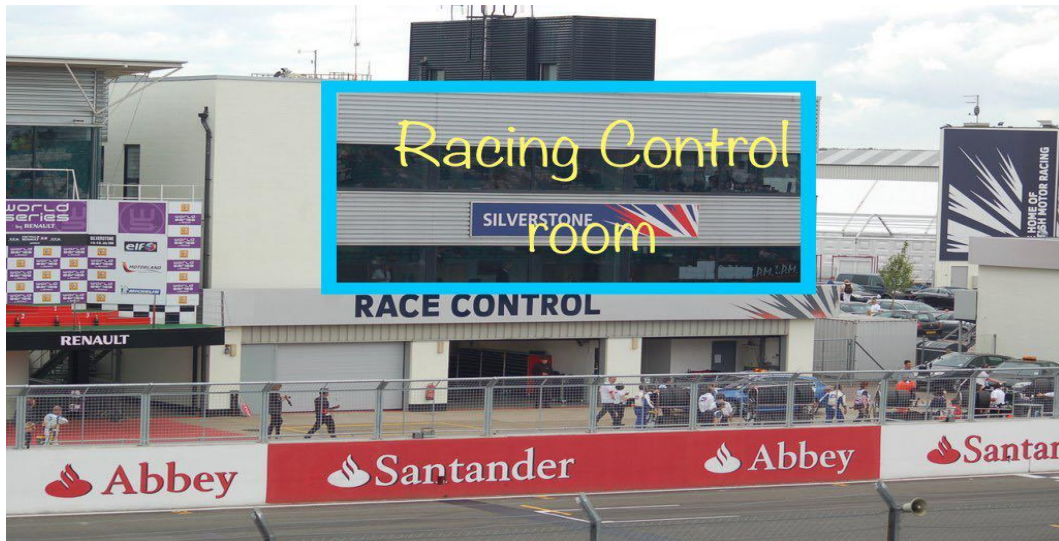
Figure 4.44: Control Room Exterior
