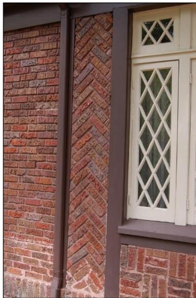
**Figure (2. 6):** Nogged brick wall
