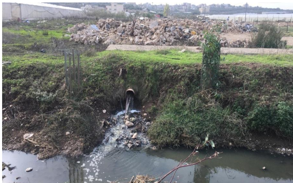
Figure 8: Outfall of sewage system forms as point source of nitrate pollution in Ash-Shaarawieh
