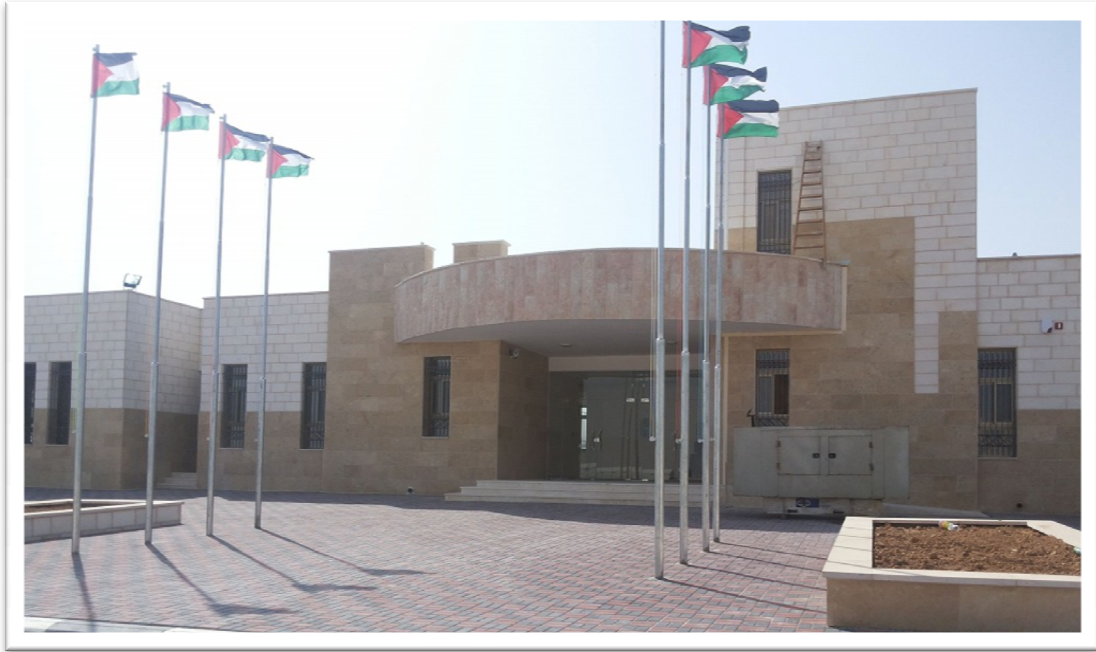
Figure (4.9): JAIP Administration building
