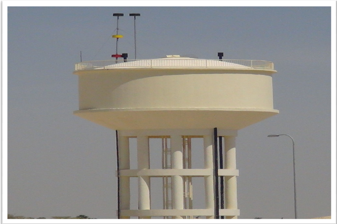
Figure (4.8): JAIP' water tank
