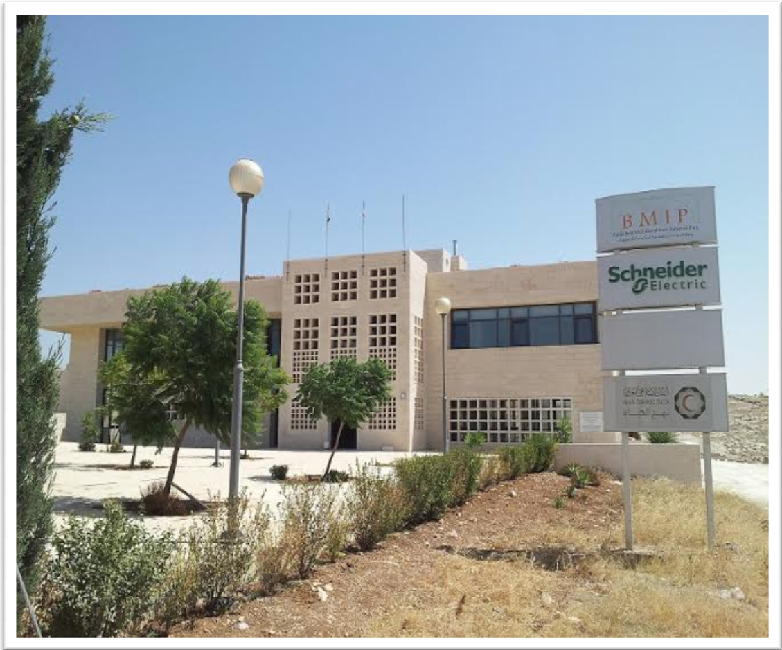
Figure (4.12): BIE's administration building
