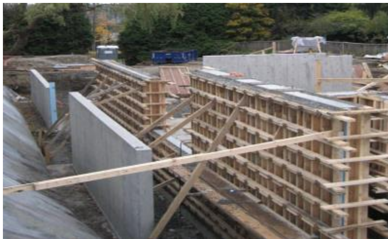
Figure: shear wall formwork
