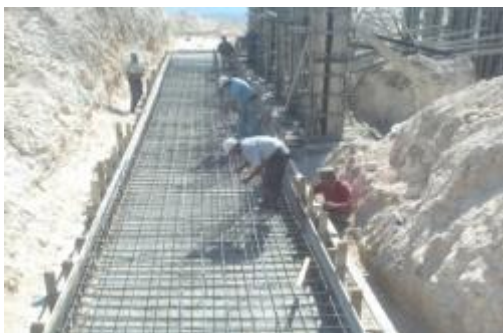
Figure 10: Wall footing.
