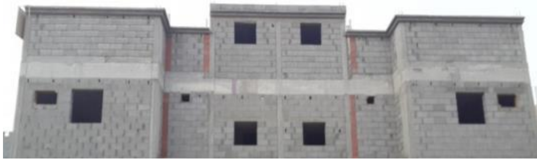
Figure 8: Non structural wall(infill wall).
