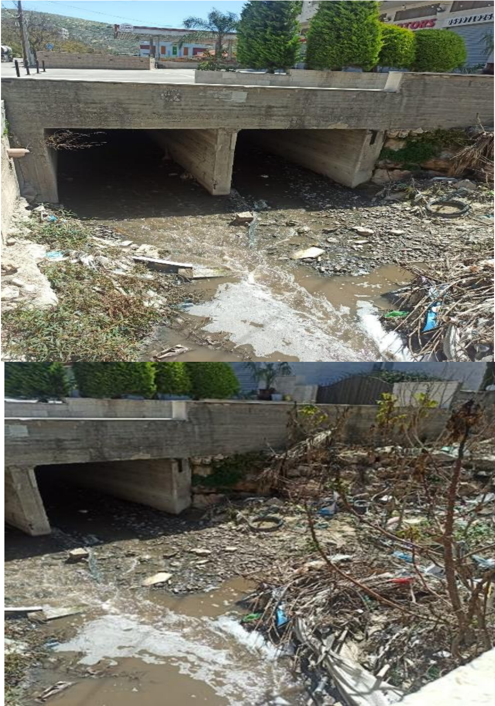
Figure A.18 Culvert in Anabta
