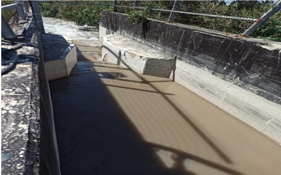
Figure A.12 Al Zeimar Catchment Sink-Partial Flume
