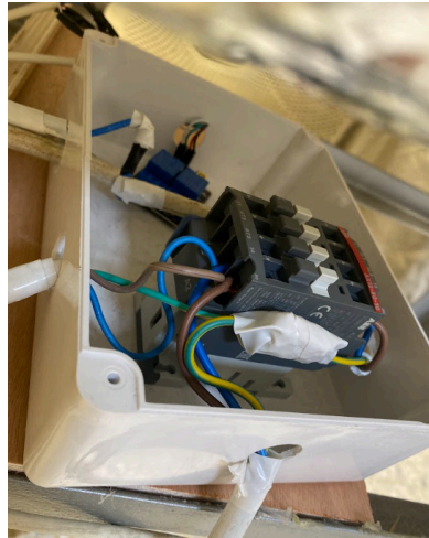
Figure 6.2.14.1: Contactor
