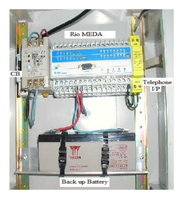
Fig. 5: Data logger Components
