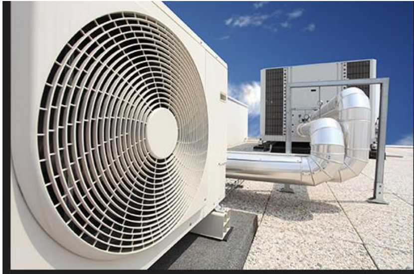
Figure 4. 77:picture for VRF system:1
