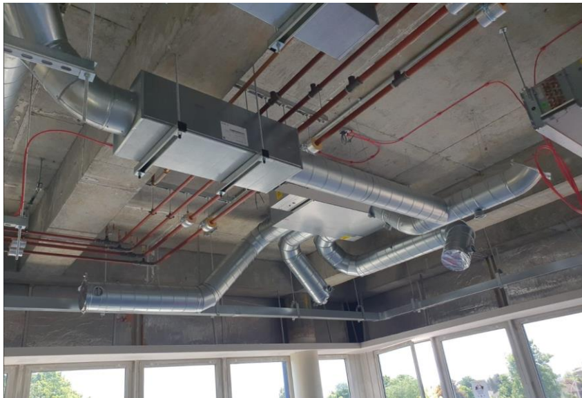
Figure 4. 78:picture for VRF system:2
