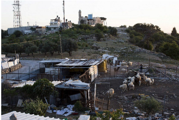
Figure 4.15: Al-Nabi Samuel buildings (Manor,2014)
