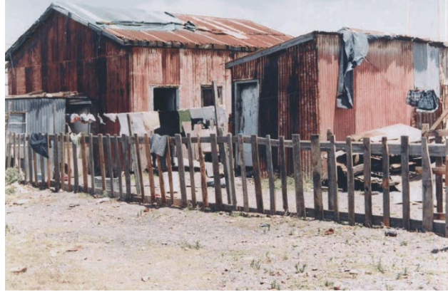
Figure 2.25: Houses at the Red Location (Msila, 2013)
