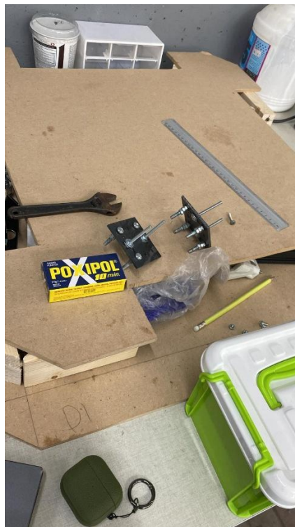
Figure 5: Assembling support structures and joints for stability.
