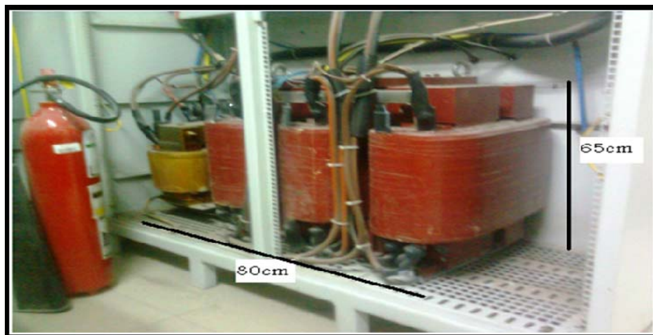
Figure (4.3): Large transformer used inside the conventional 100kVA UPS
