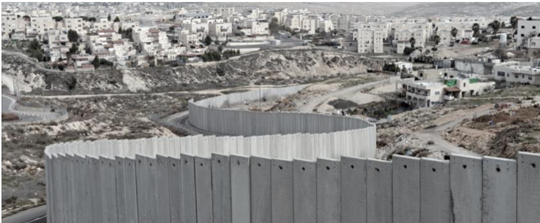
Figure (4.3): The wall is made up of 8–9-meter concrete slabs (Source: OCHA, 2007).
