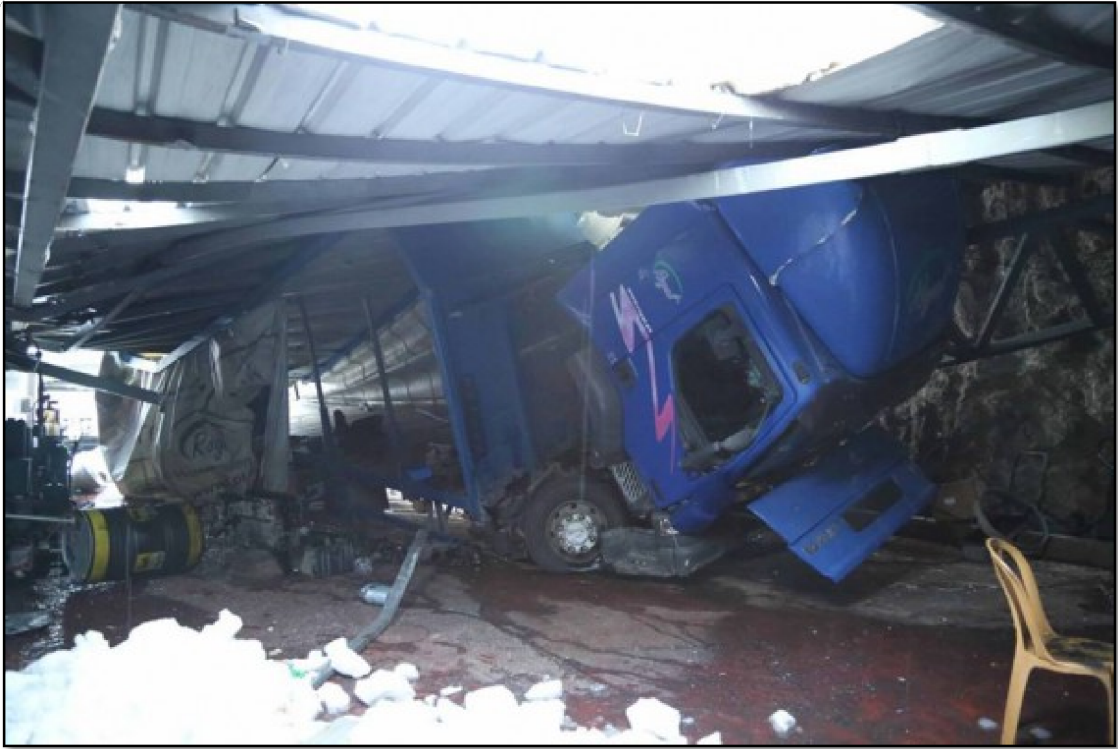
Figure B.2 Snow fall adverse effect on Royal company truss
