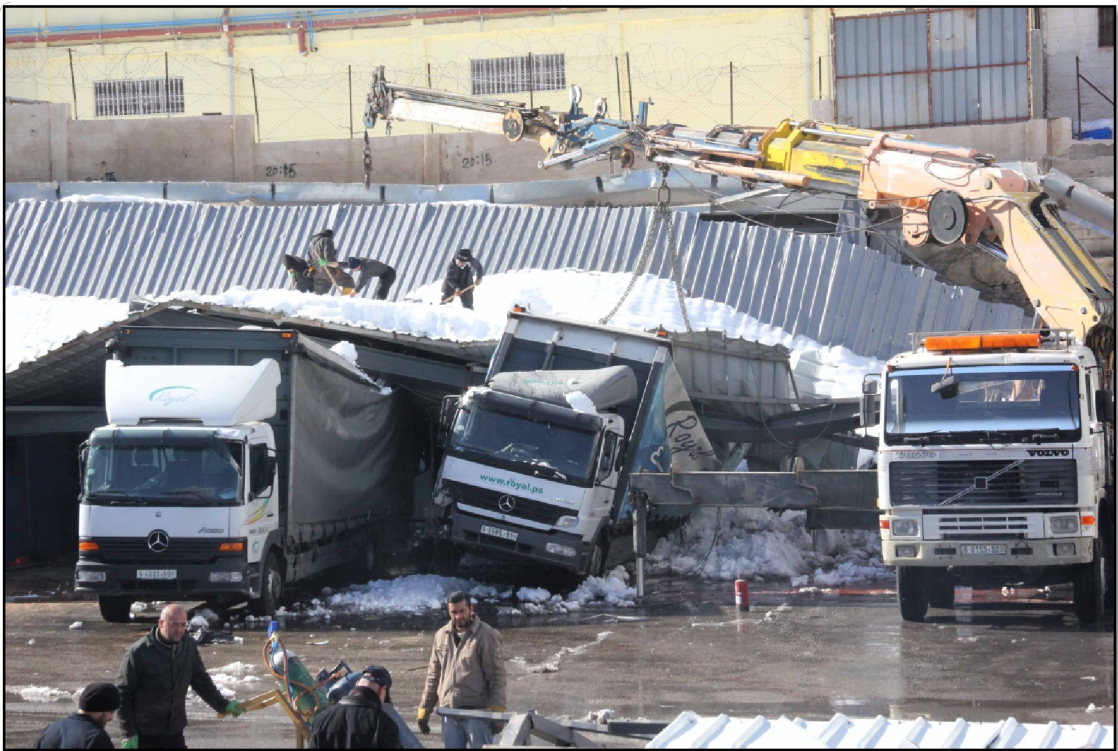
Figure B.3 Snow fall adverse effect on Royal company truss
