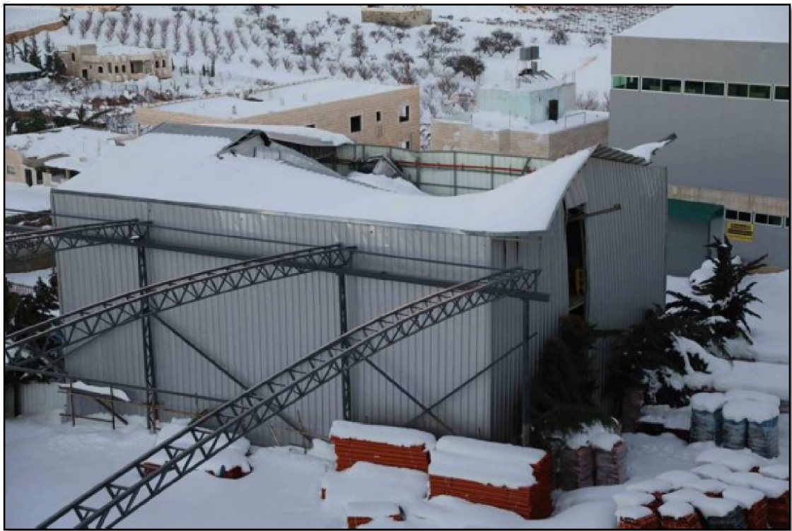
Figure B.1 Snow fall adverse effect on Royal company truss
