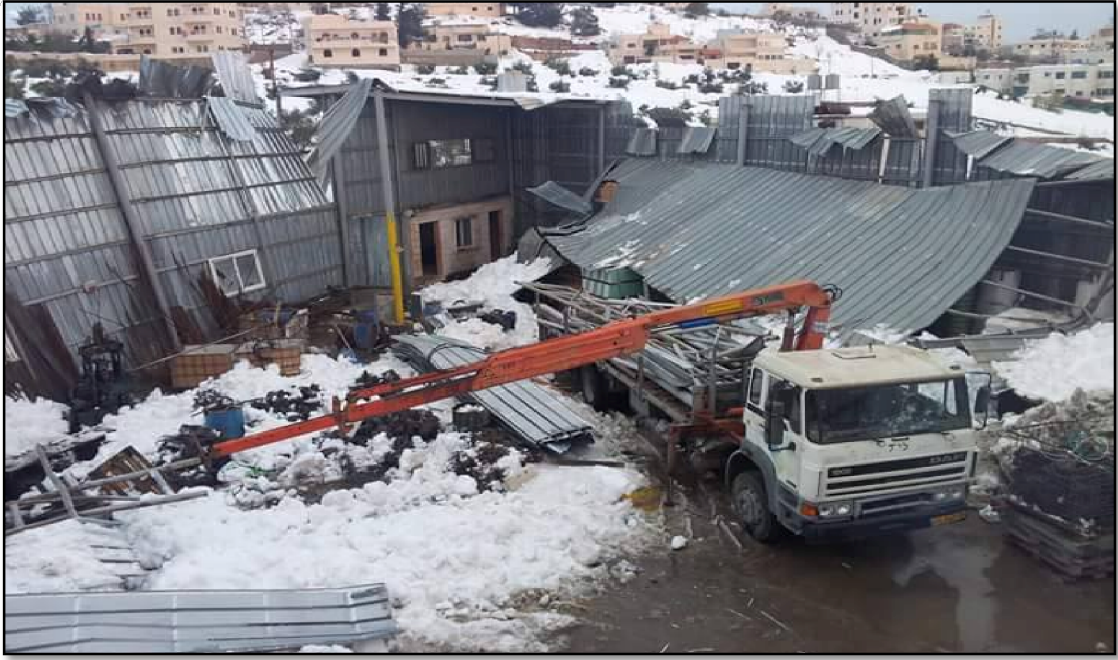
Figure B.5 Snow fall adverse effect on Shahatet company truss
