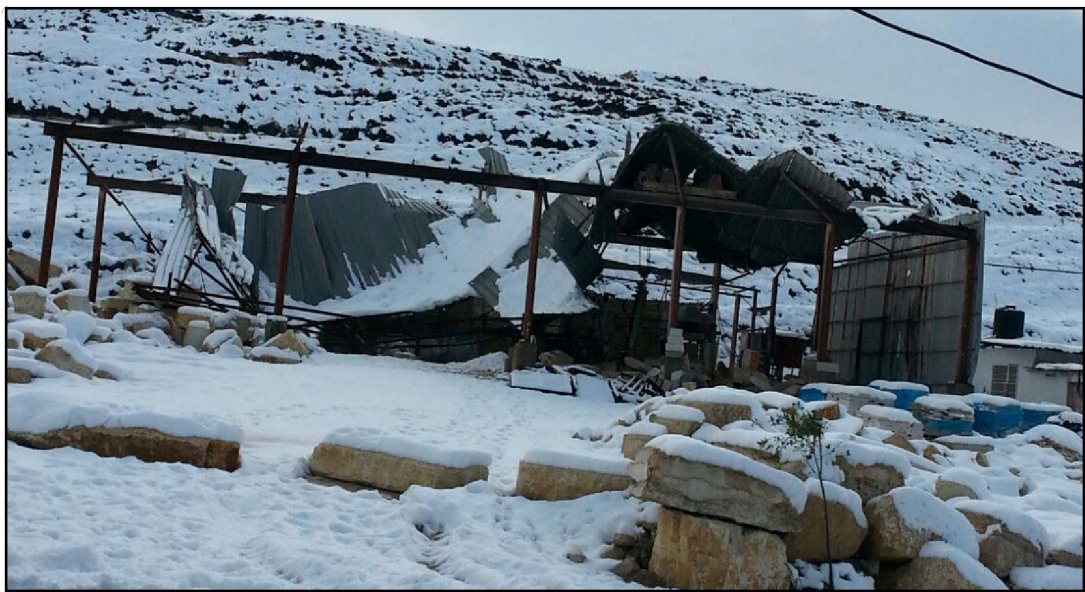
Figure (4.1): Snow fall effects on Jamaeen stone cut truss.
