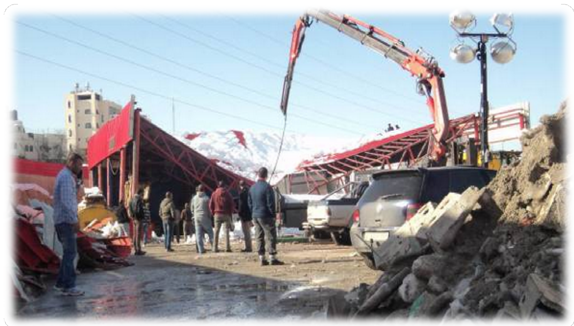
Figure (2.18): Snow fall effects on Al Mahaba Company.
