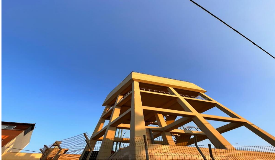
Figure 12 Yasid elevated tank
