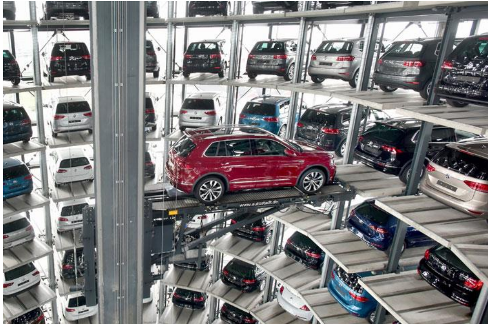
A Large Fully Automated Parking System
