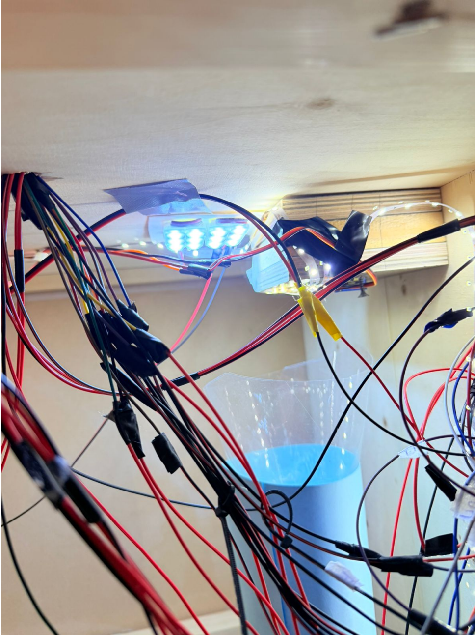
Figure 3.7: Fixed LED lighting at the inspection station.
