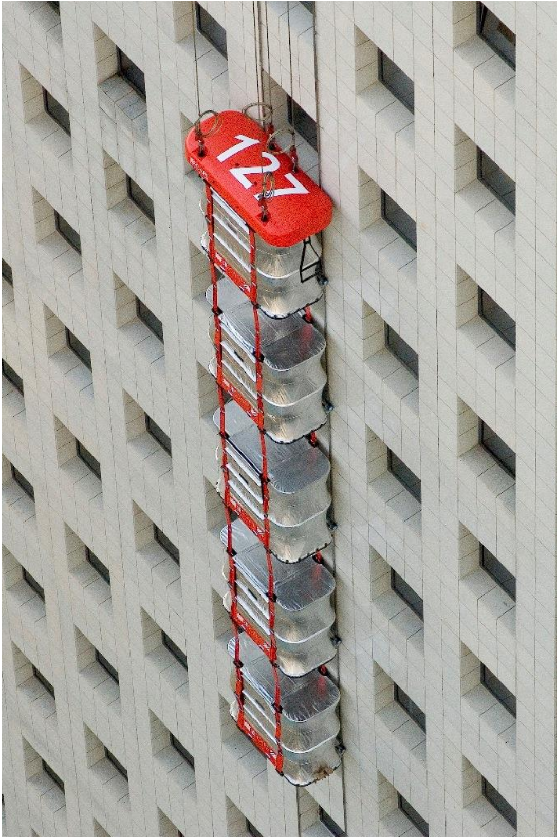
Figure 311 emergency elevator (escape and rescue system, n.d.)
