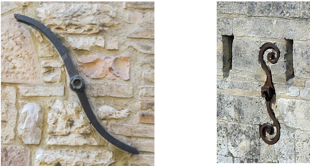
Figure (5.15): Ties of Masonry Buildings
