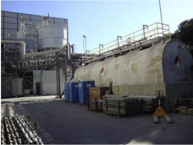
Figure (2.13): Ammonia Tanks Installation in WtE Plants (Source: Rogoff and Screve, 2011).
