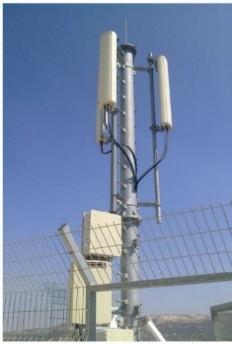
Figure 3.1: Radio Site the RBS is in the shelter
