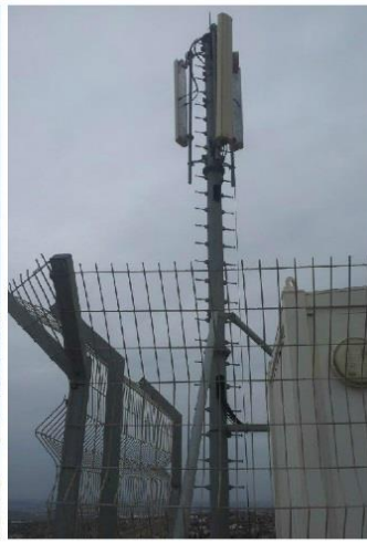
Figure 3.1: Radio Site the RBS is in the shelter
