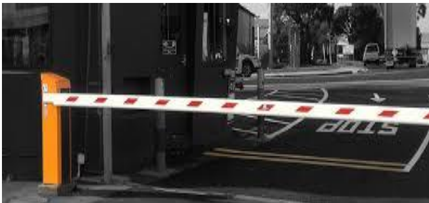
Figure 6.5.a: Automated Entry Gates
