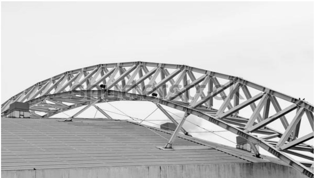
Figure 7.d: Tied Arch Truss
