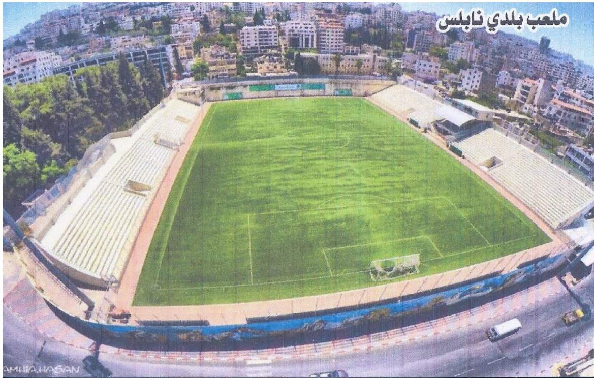
Figure 1.1.2.a: Nablus Municipal Stadium
