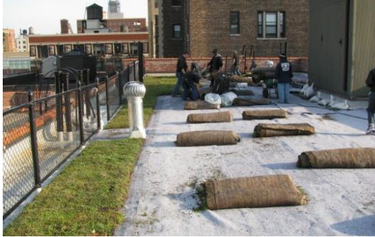
Fig. 12 Mat based system Source: (Dorsey, 2013)
