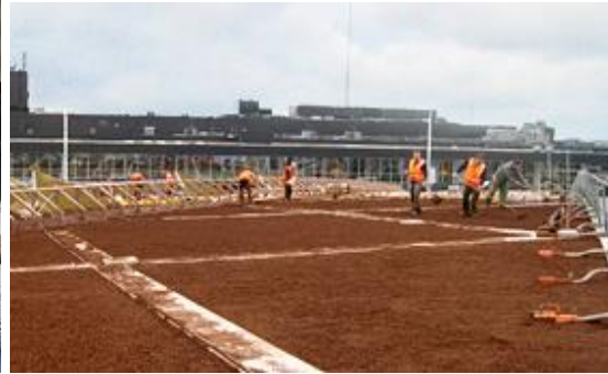
Fig. 13 Substrate based system Source: (“Green Roof Report | ZinCo,” 2012)
