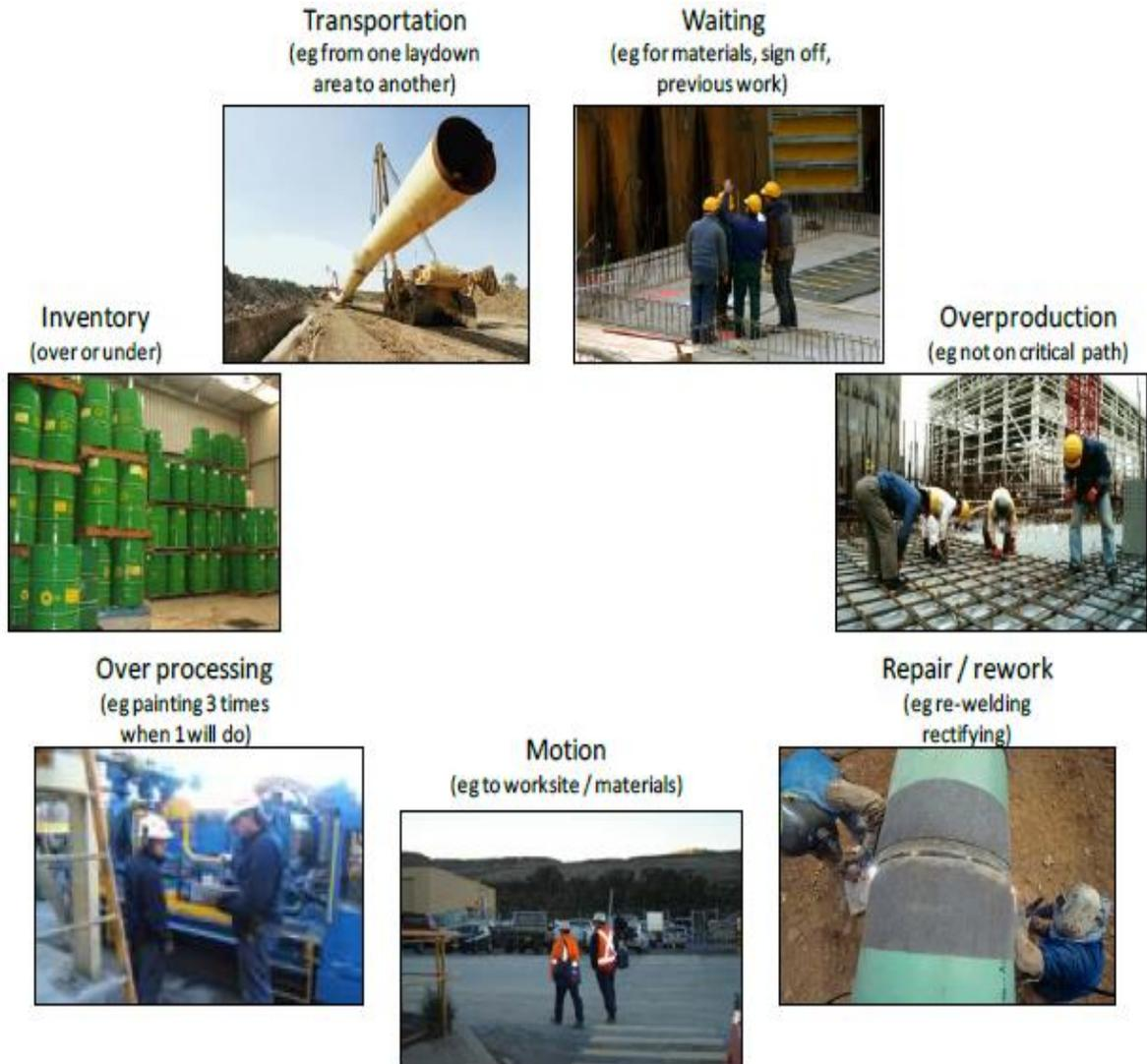
**Figure (3:1) :** Seven waste in construction
