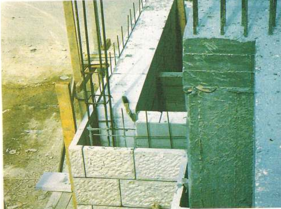
Figure (2.16): Exterior wall in which stone units are built backed with lightweight blocks.
