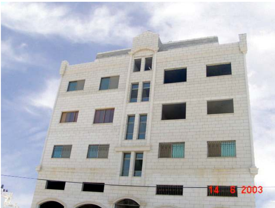
Figure (2.10): Building with cast stone
