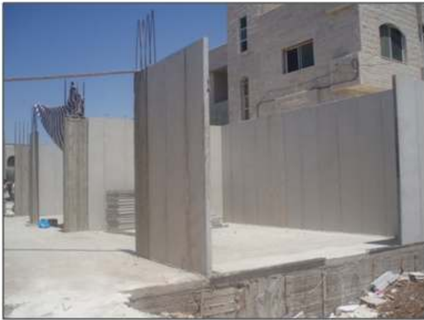
Figure (2.7): External walls and internal walls from concrete wall panels. Source: (Jayyousi, 2011).
