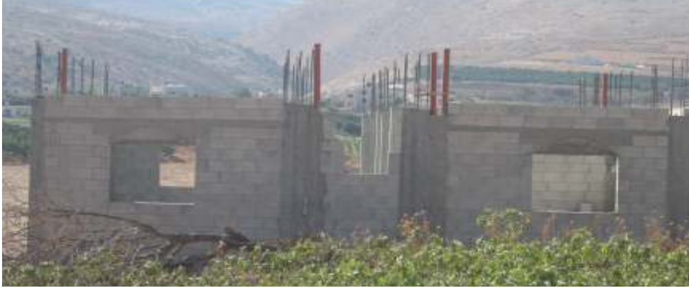
Figure (2.17): Exterior walls built from concrete blocks.
