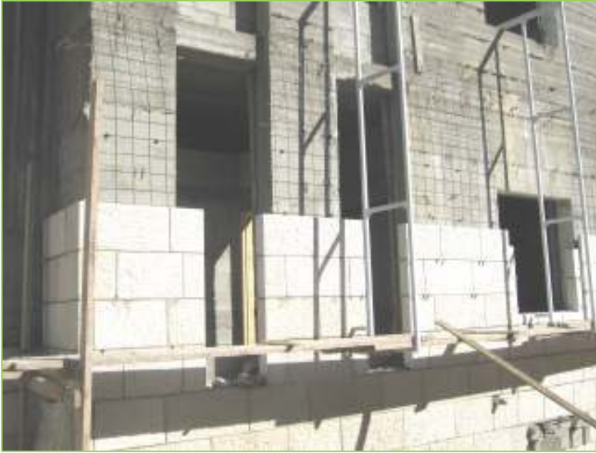
Figure (2.9): External reinforced concrete walls with natural stone cladding.
