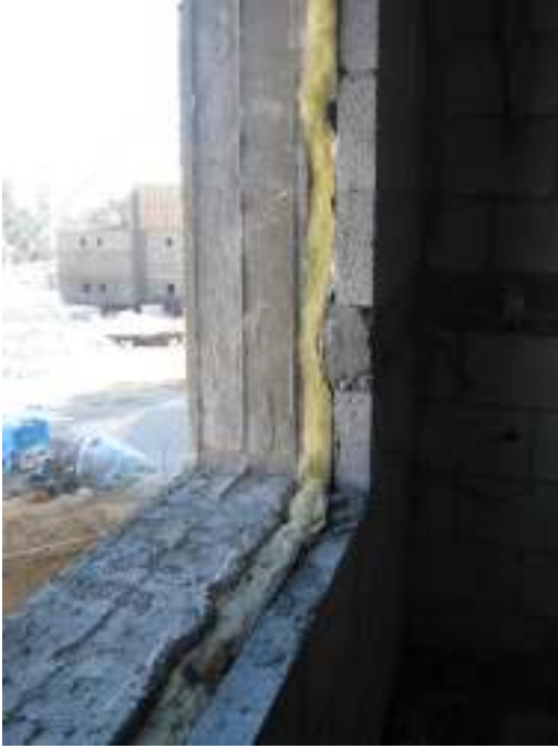
Figure (2.14): Insulating material between the two walls
