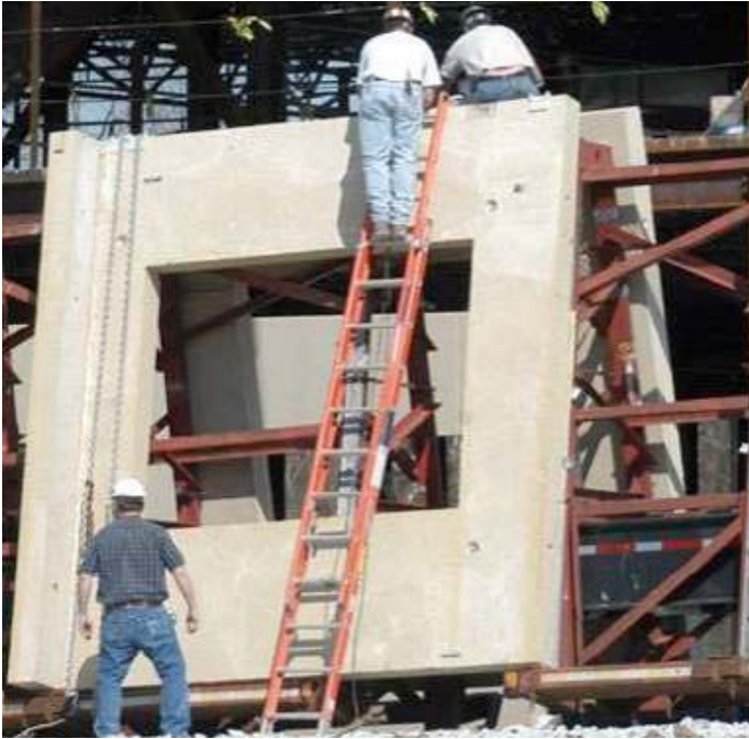
Figure (2.6): Precast concrete wall panels.
