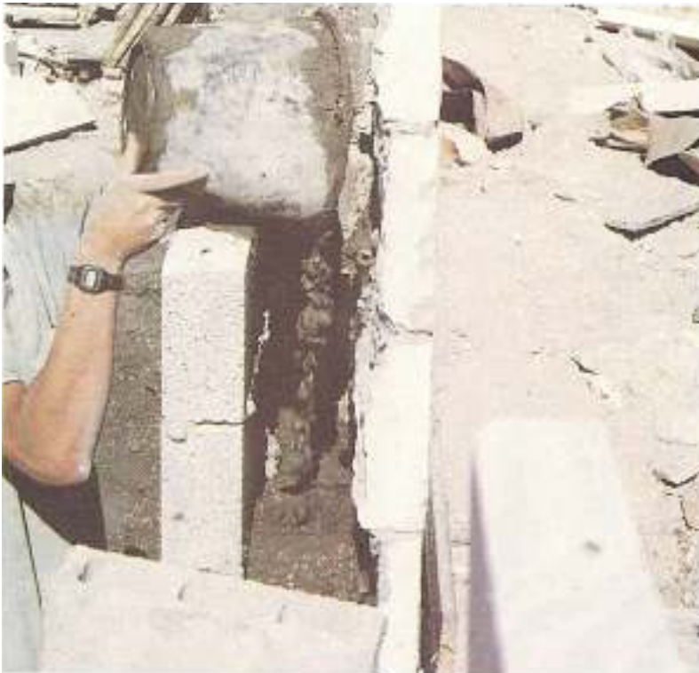
Figure (2.12): Exterior walls built from concrete, stone and concrete block.
