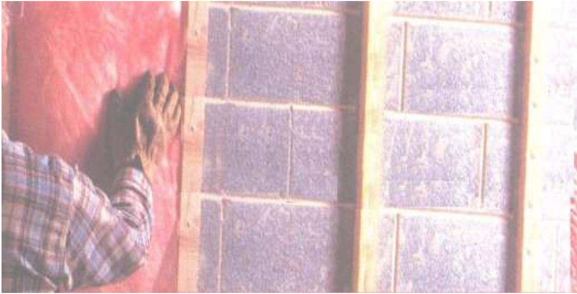
Figure (5.2): Mineral fibers are fixed between the wood studs.
