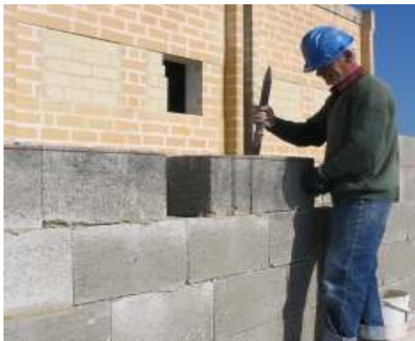
Figure (2.8): Concrete blocks wall
