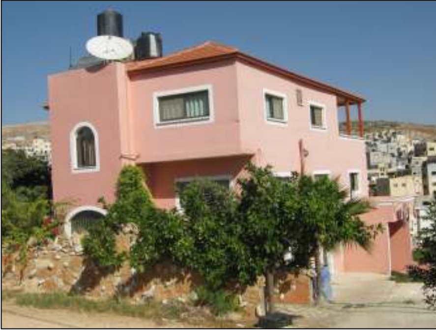
Figure (2.2): Concrete hollow block building. Source: (The researcher, 2010)
