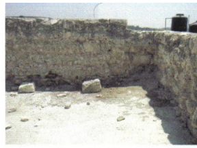
Single layer stone facing wall
