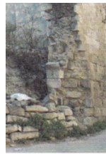
Double layer stone facing wall
