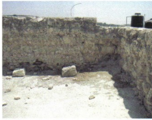
Single layer stone facing wall
