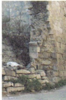
Double layer stone facing wall
