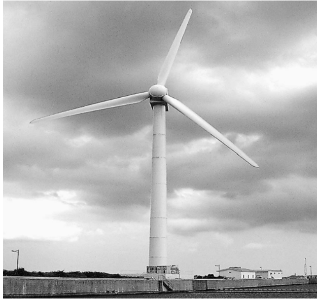
Figure (3.4): 3-blade HAWT, 2 MW, Okinawa, New Energy Development Company-(Japan).
