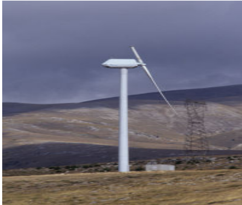
Figure(3.2): 1-blade HAWT from Riva Calzoni, central Italy, 1998.
