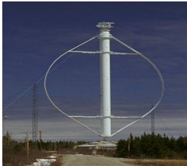
Figure (3.6): A 4 MW, Darrieus-type VAWT, Cap Chat, Quebec, late 1990s.
