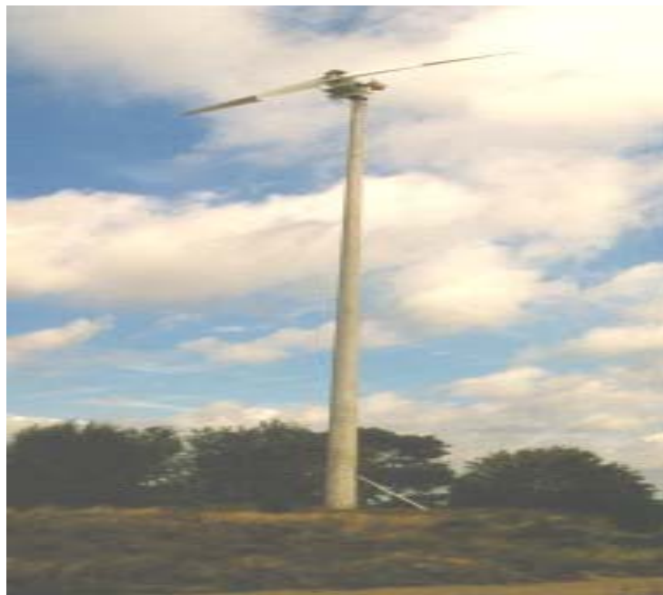
Figure(3.3): 2-blade HAWT, 30 kW, Pitch Wind Systems AB Company (Sweden).
