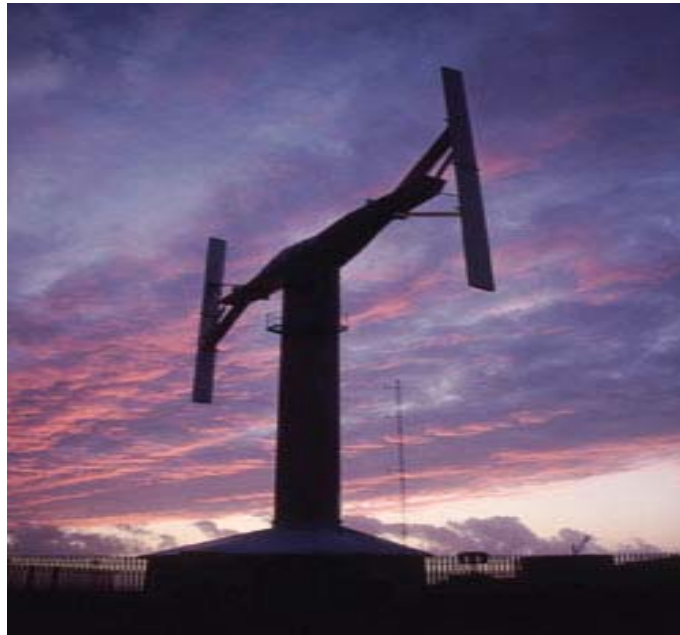
Figure (3.7): A H- type VAWT built in Wales, rated power 130 kW.
