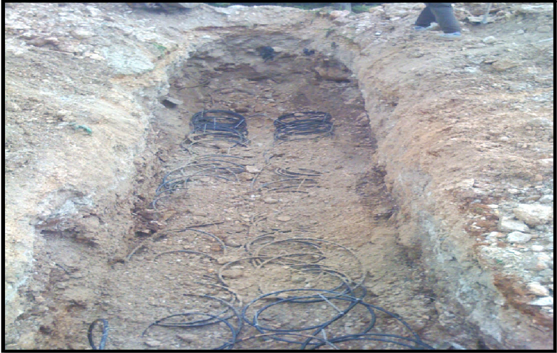
Figure (5.3) Trench after finalizing the pipes and backfilling
