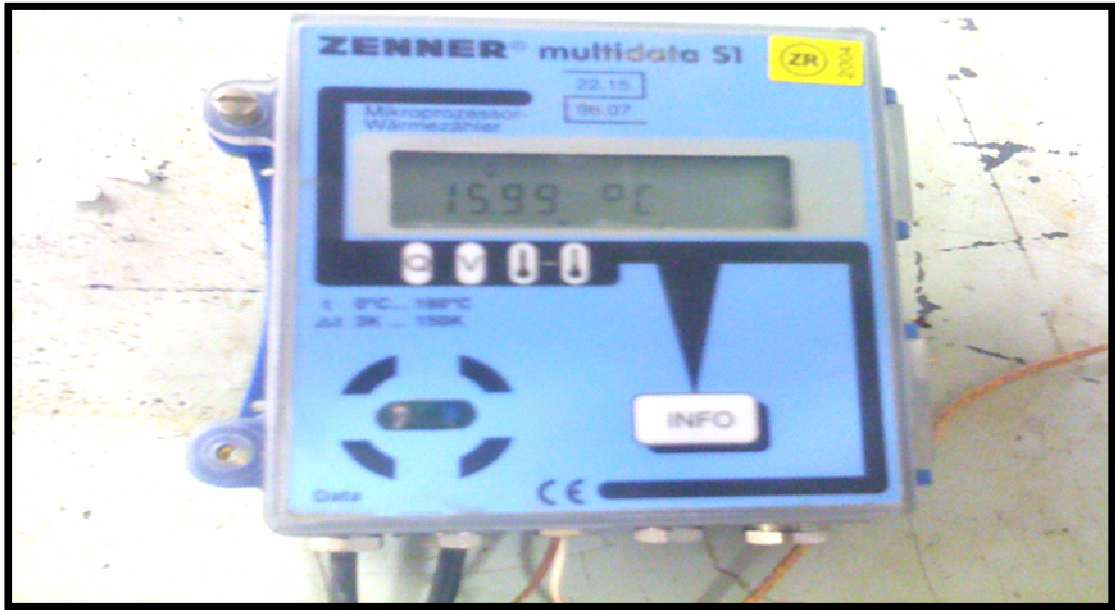
Figure (5.7) Multidata S1 logger heat meter type Zinner
