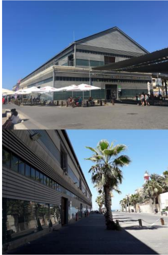
Figure 18 Warehouse 1. A) The southern entrance to the building (top). B) The northern façade. Source: Nufar Avni
