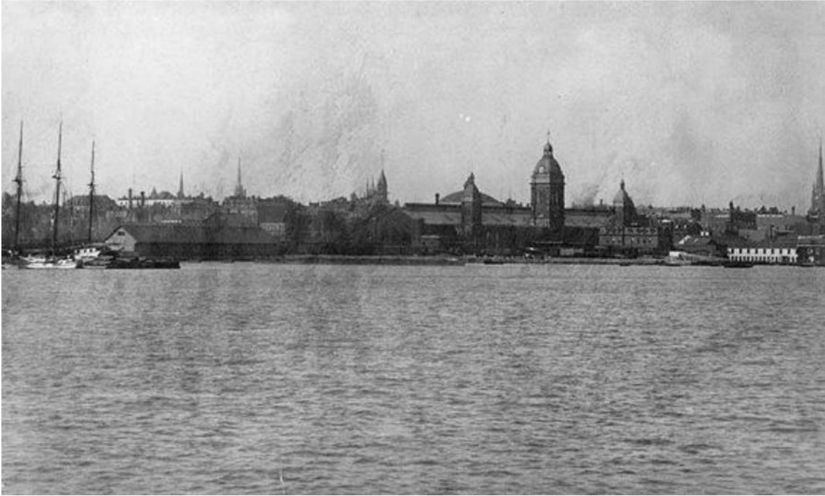
Figure 9 fToronto Harbor 1870, Source: Flack, 2011.
