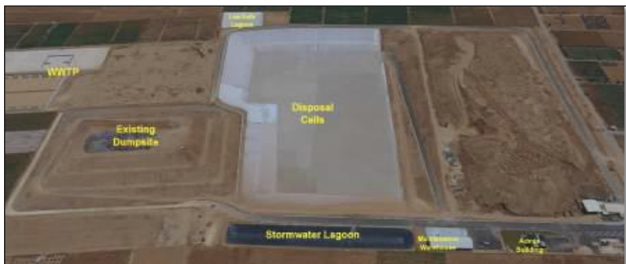
Figure 18 Al-Fukhary Sanitary Landfill and Existing Dumpsite
