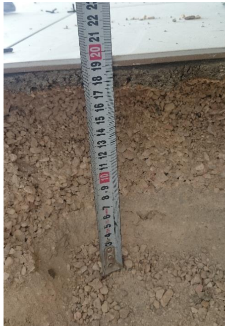
Figure 1.1: 20cm thick filling material overlying 25cm ribbed slab with hidden beams
