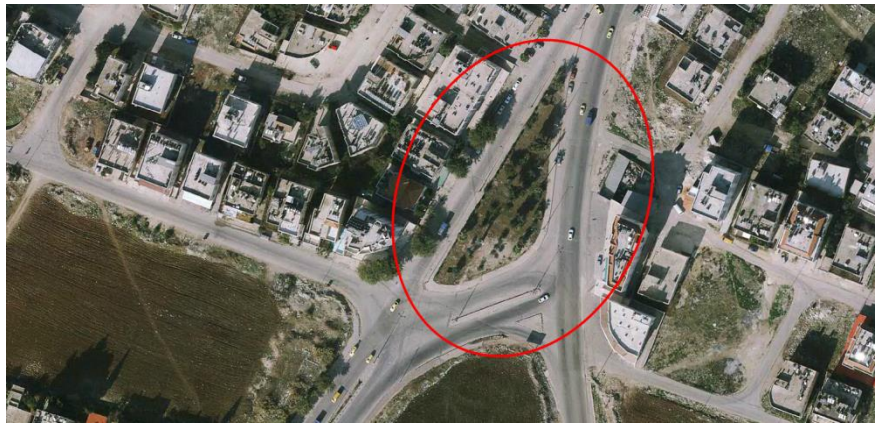
Location of roundabout
