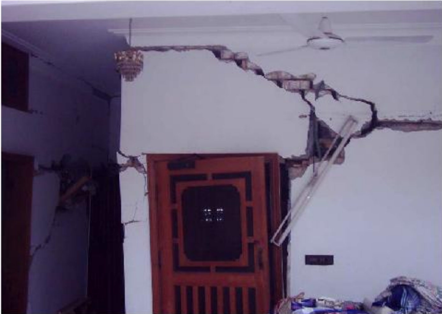
Figure 5: Severely damaged unreinforced brick masonry wall in Muzaffarabad
