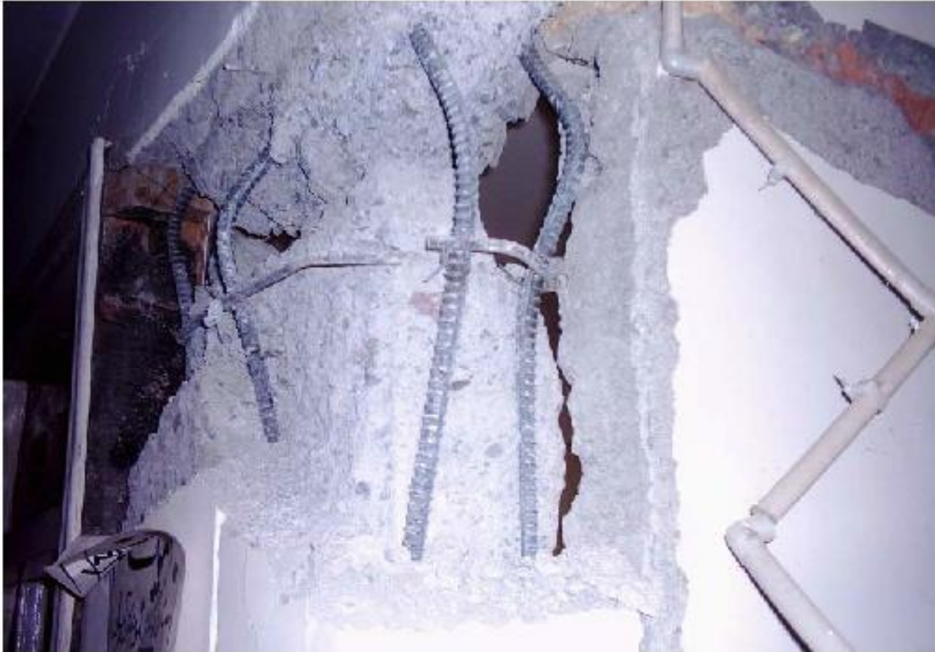
Figure 7: Formation of plastic hinge in the column near the beam-column joint in a hospital building in Mansehra
